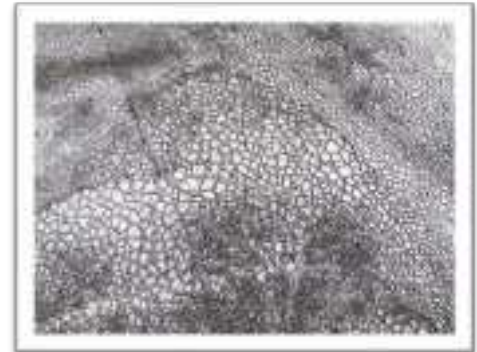
Figure 13: "Alligatored" roofing condition
