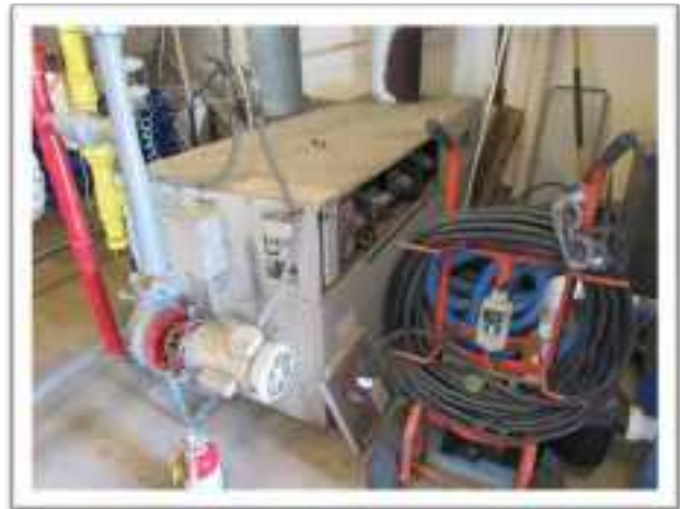
Figure 57: Pool water heater
