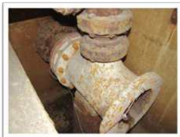
Figure 54: Corroded piping
