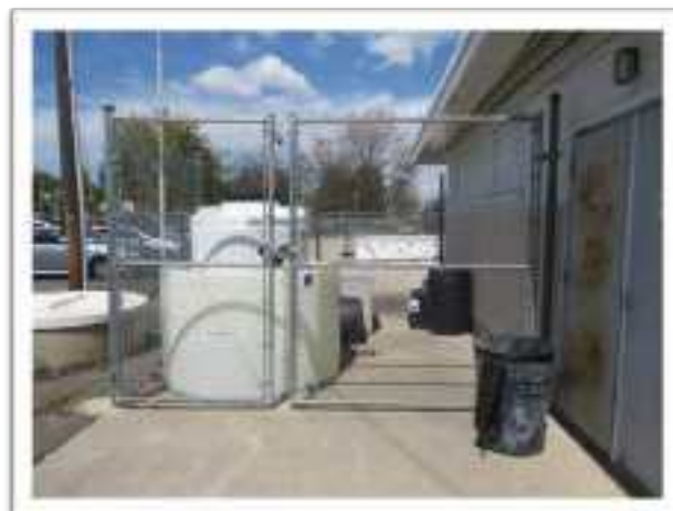
Figure 55: Chlorine storage tank
