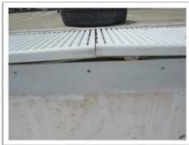
Figure 48: PVC gutter
