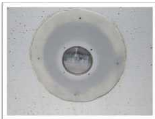
Figure 49: Underwater lights in wall
